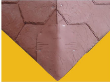
Picture 2: Install the first piece at the bottom of the hip. Cut the top shingle to line up with the other shingles. Mold shingle to the shape of the hip.
